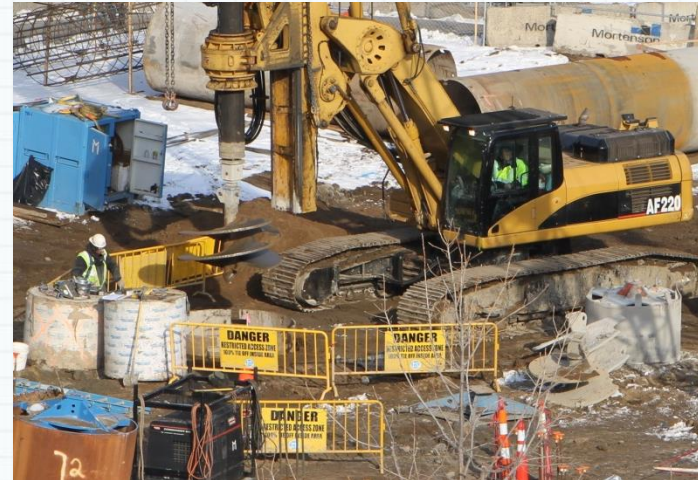
Auger Cast Pile Placement
